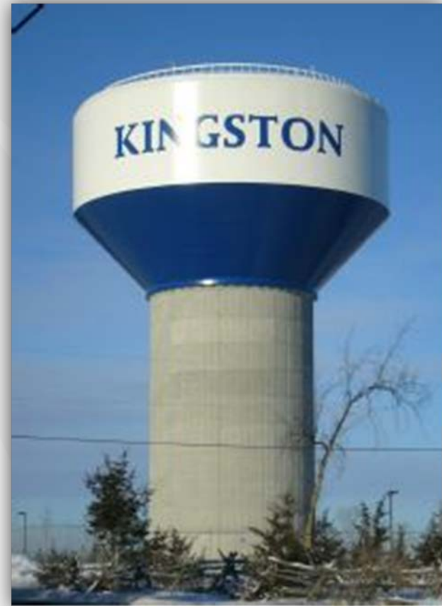
Creekford Road Elevated Tower
