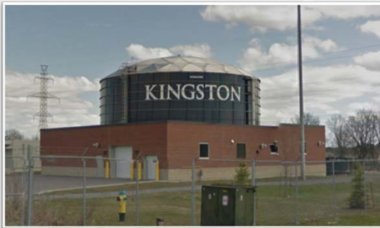
O'Connor Drive Reservoir and Booster Station
